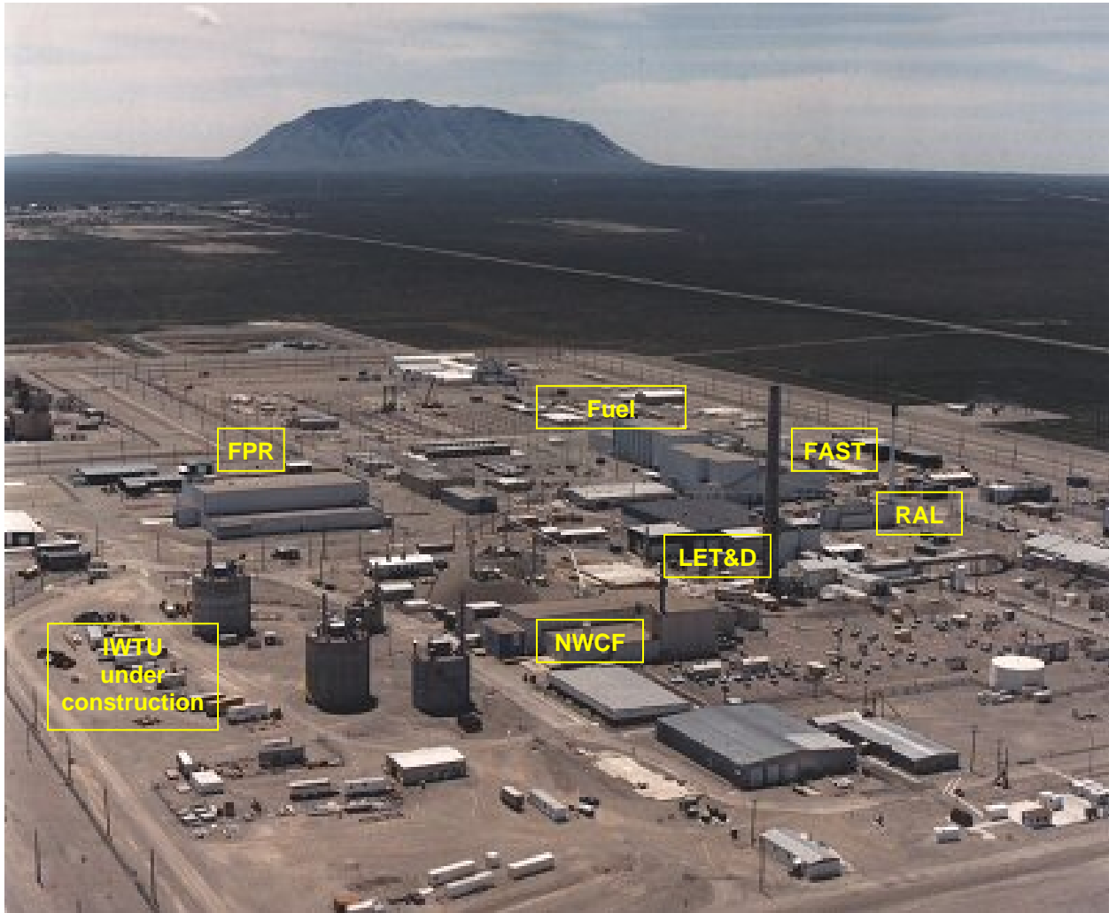
Figure A1-1. Aerial view of INTEC at INL. Labeled facilities proposed for supporting the AFCF mission are described in the text.
